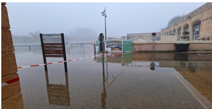
Parking Saint Pierre – quai de Verdun submergé
